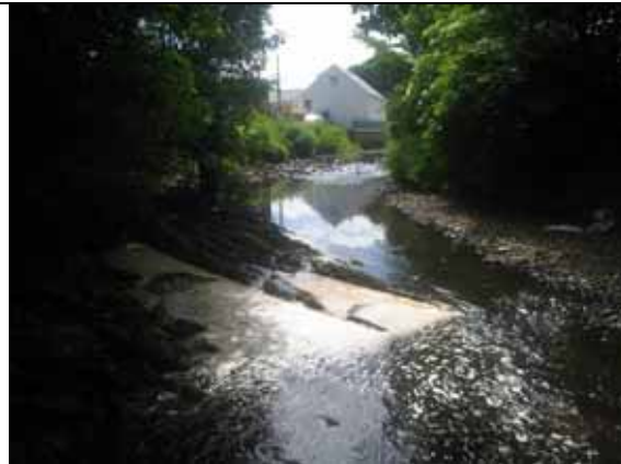
Site 2. Galey River. Downstream of Athea Bridge for c.150m. Generally unsuitable habitat due to heavy siltation and filamentous algal growth. No evidence of mussels. Raw sewage entering river from pipe.
