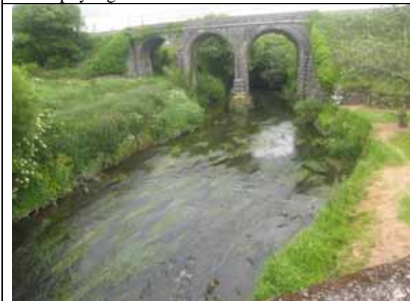
Site 5. River Maine. View upstream from Curran's Bridge. Searched upstream from Curran's Bridge to Q 93908 06610. Total length of stretch searched 205m. Habitat appears suitable but heavy macrophyte growth, filamentous algal growth, and heavy siltation covering substrate. No evidence of mussels.
