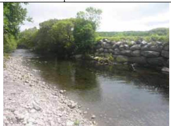
Site 9. Adrigole River. Upstream of Adrigole Bridge. Mostly unsuitable habitat (bedrock, mobile boulders) up to V 81226 50625. Abundant mussels under western bank upstream of bend at V 81185 50724 and for 50m upstream, then absent. Major bank protection works probably damaged population at this location.
